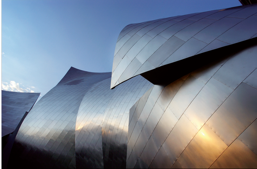
Figure 1.7. Titanium-clad roof, Richard B. Fisher Center for the Performing Arts, Bard College, Annandale-on-Hudson, New York. Photograph by Andy Wainwright, 2011.
